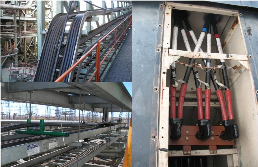
Structural steel and electrical cable tray installation. 18,000 feet of 1000 MCM cable installed at heights ranging from 13' to 87'. Arizona Public Service (owner) supplied the materials.
